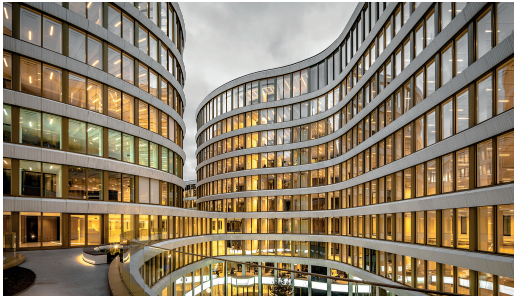
BNP Paribas Fortis headquarters in Brussels, delivered in November 2021 by Eiffage Benelux
