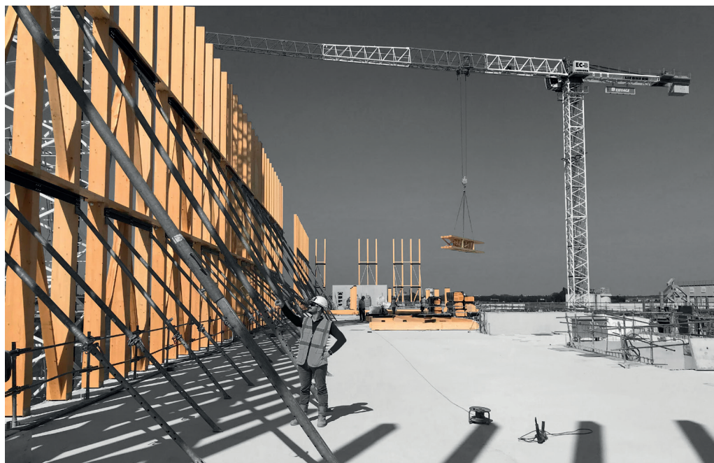
Worksite at IN'CUBE, the future Danone research and development centre (Essonne)
